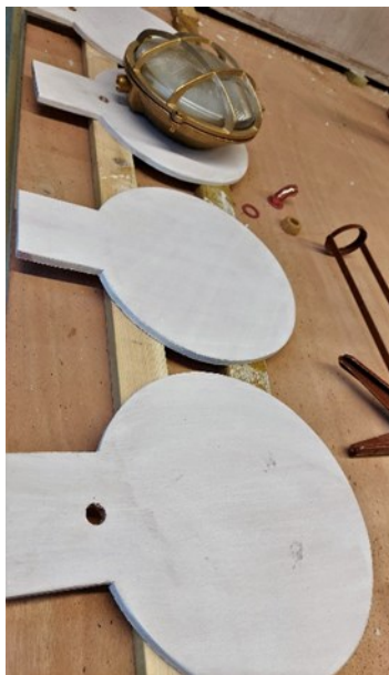
Above left: Backing boards for lighting units and Above right: Lighting unit loose assembled at the Shed (at the Pier) (Photos - Alan Titheridge)
